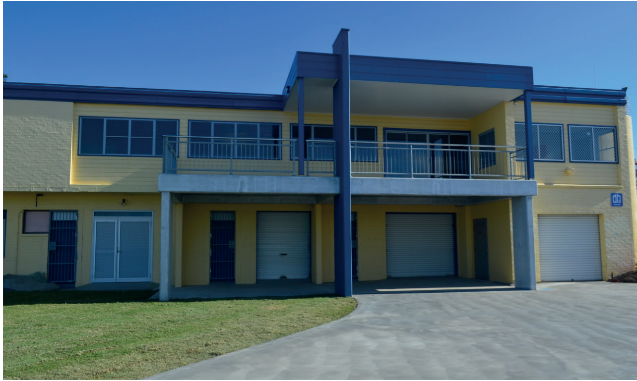
Newly Finished Renovated Surf Club.
